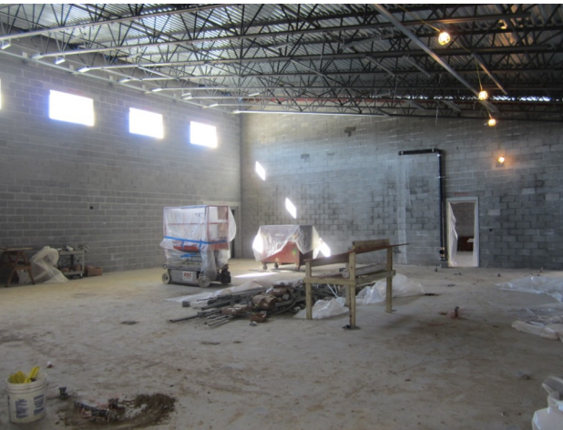
Top Left: The new Enforcement Bureau is taking shape. It will house the Street Operations Unit and a new muster room.
