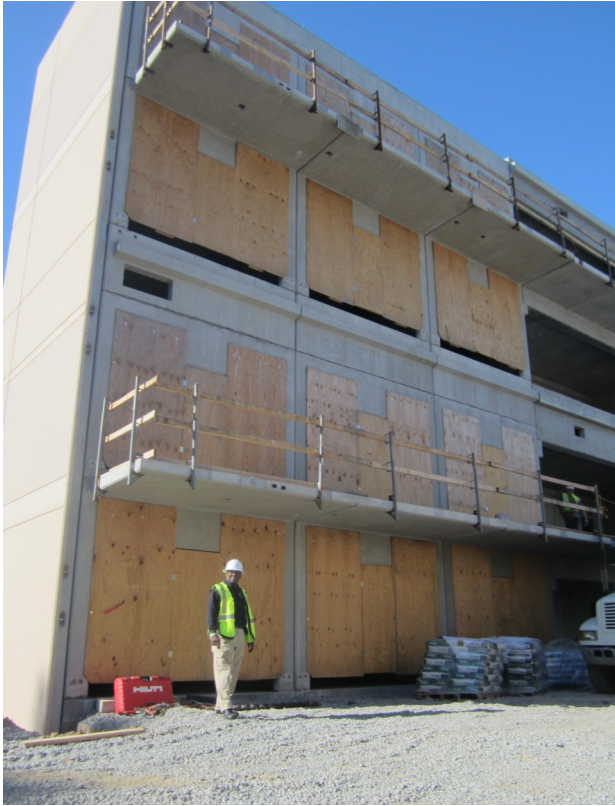
Above: Cpl. Smith is dwarfed by the new four-story inmate housing tower. The towers stand 45 feet high.
