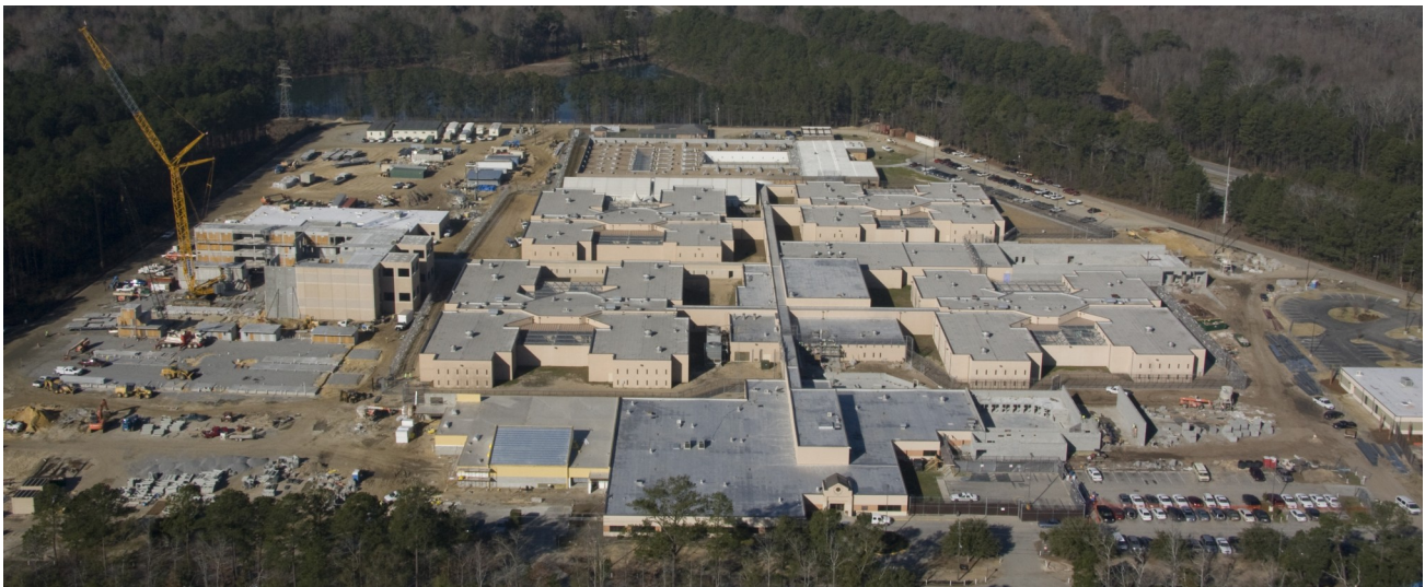
Above: The Detention Center Expansion Project is moving full steam ahead. This massive construction project will nearly double the inmate housing capacity and create larger workspaces for street operations, booking, medical, programs, the kitchen, warehouse and administration.
